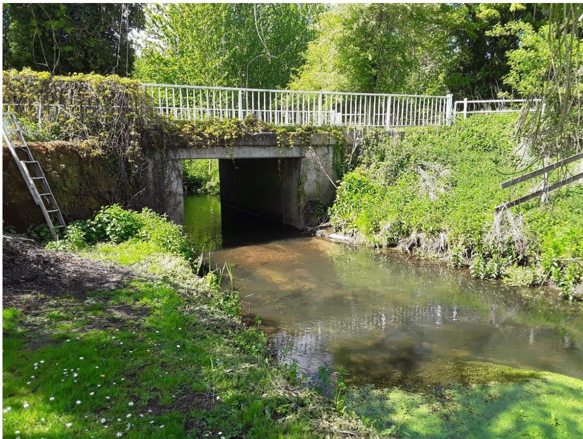
Caption 3.3 - Blois Bridge, looking upstream.
